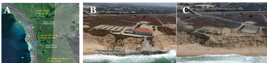
Figure 14 (left): Examples of some adaptation success stories, such as: Hwy 1 Piedras Blancas Realignment (A); and preventing further coastal erosion by removing Fort Ord (B-before removal, C-after removal).
